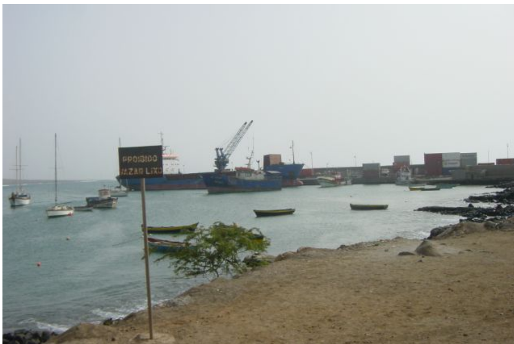
Figure 2-1 Palmeira Port seen from the water front at Palmeira village
