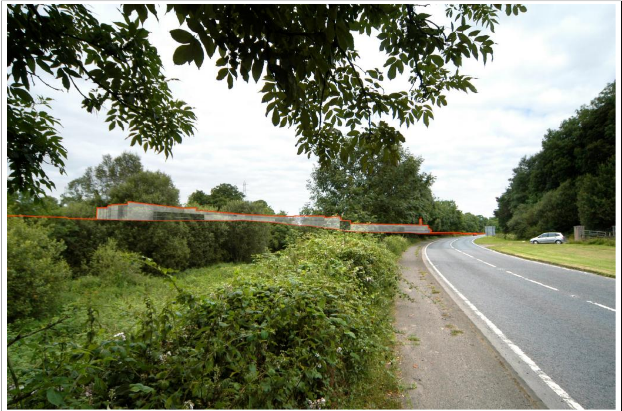
View 1 – A32 Irvinestown Road Looking North. Hospital buildings screened by trees – outlined in red
