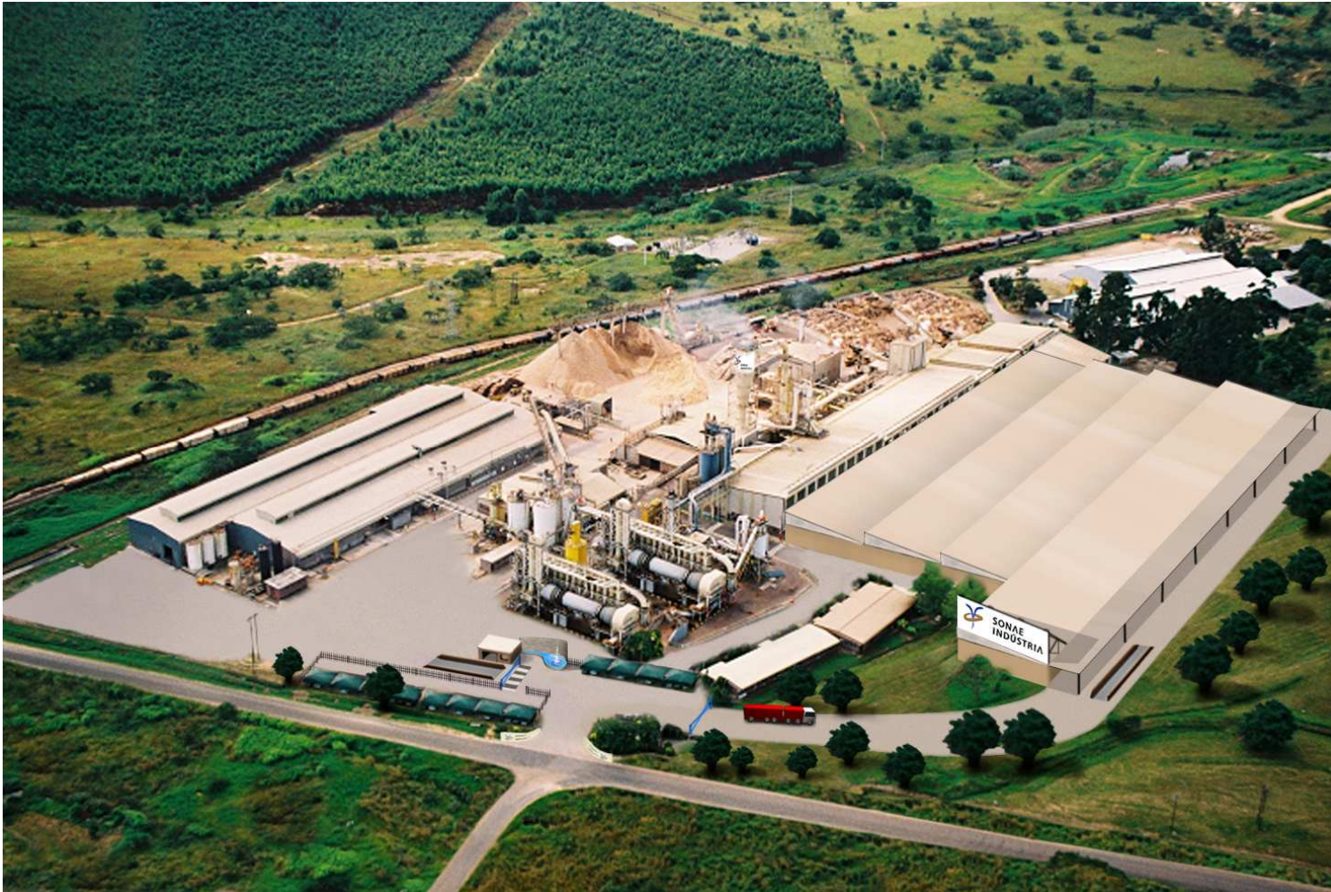
Photograph 3: Aerial View of Proposed Changes (Two driers are shown above. The old drier will be demolished once the new drier is built).
