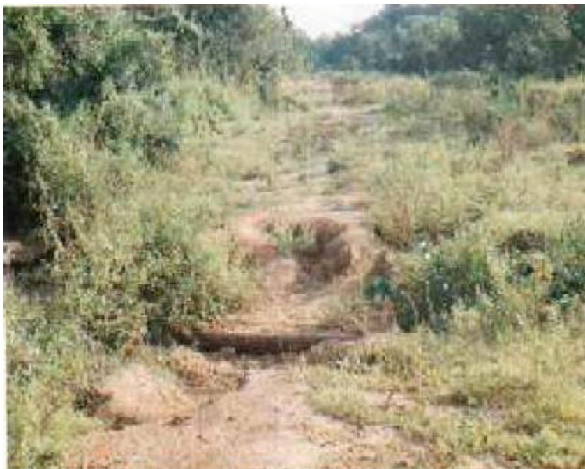
Plate 4.5: Exposed Existing Pipeline along the ROW
