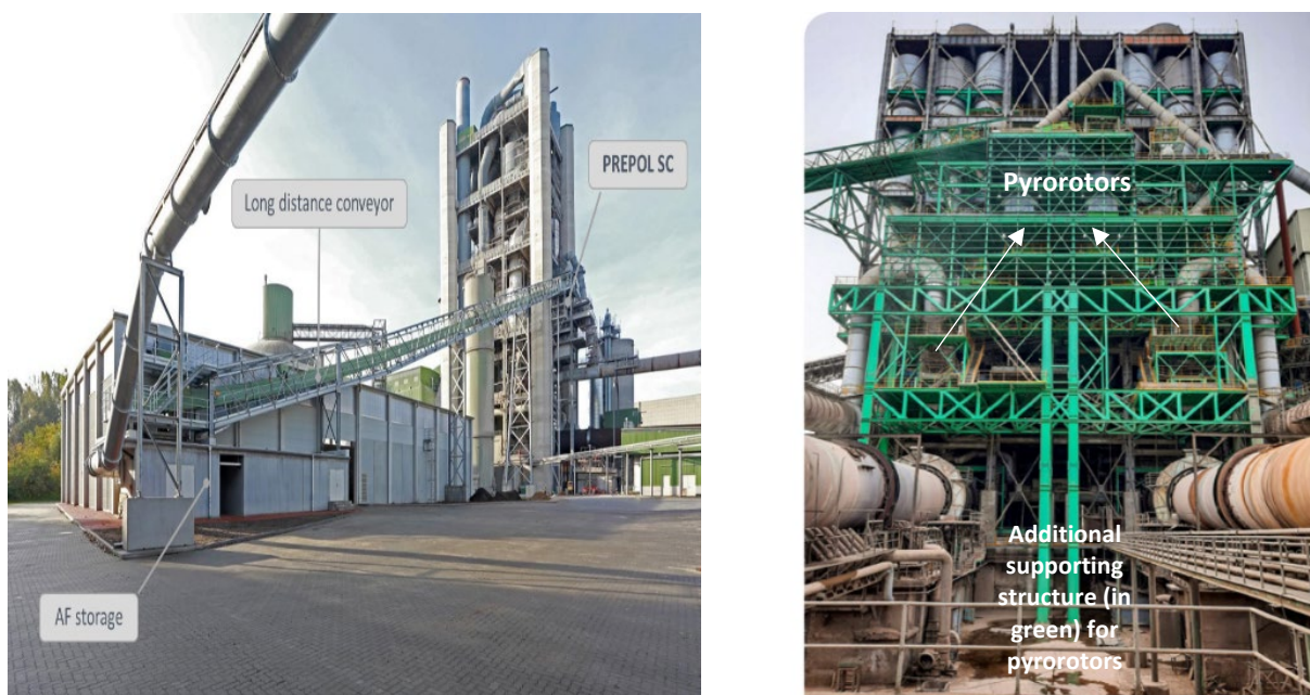
Figure 34: Left: Installation of Prepol SC by Thyssenkrupp in a cement plant in Germany. Right: Installation of Pyrrotor by KHD in a cement plant in South Korea
