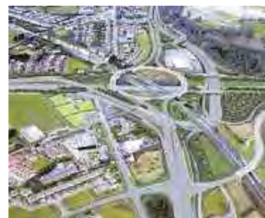
Upgrading of M50, Dublin
