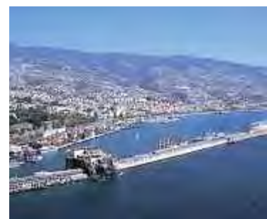
Upgrading of port infrastructure, Madeira
