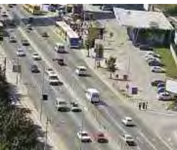
Rehabilitation of road network, Serbia
