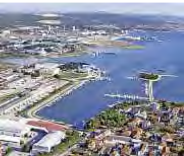
Port infrastructure, Croatia
