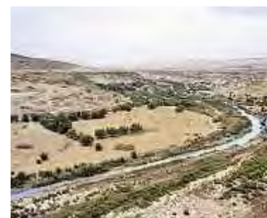
Construction of Fez-Oujda motorway, Morocco
