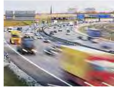
Motorway bypass, Thuringia
