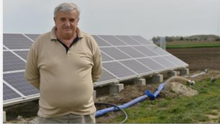
Client from Begeč – Solar system for irrigation, capacity 7 kW for 6 ha
