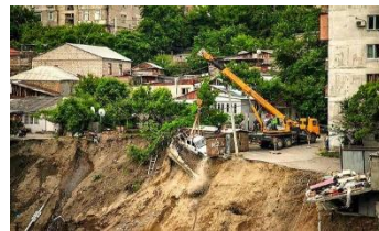
Upgrade of Municipal Infrastructure
