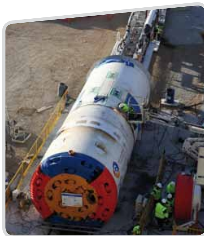
INELFE Interconnexion France, Spain CAB disbursement: EUR 15m
