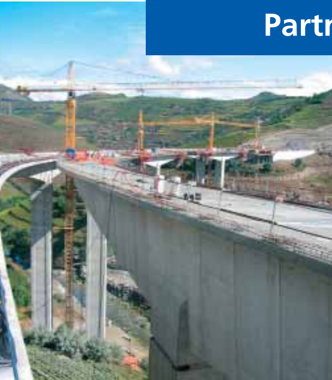
Scut Interior Norte, Portugal
