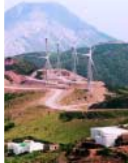
Wind farm, Tetouan - Morocco
