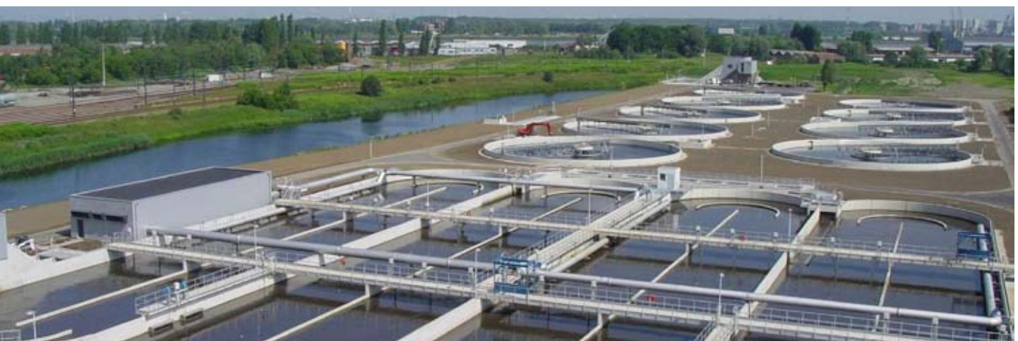
Wastewater Treatment - Belgium
