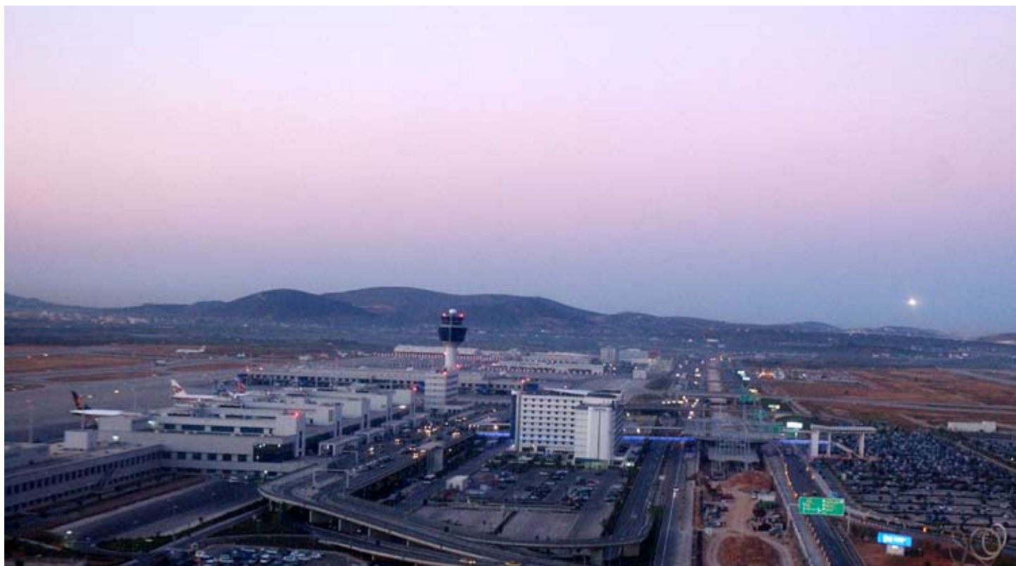
New Athens International Airport - Greece
