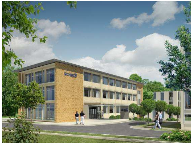
Figure 13: View of the Kiekert building, Heiligenhaus
