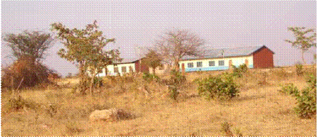
Figure 6-4: Affected Secondary School (Tumuli)
