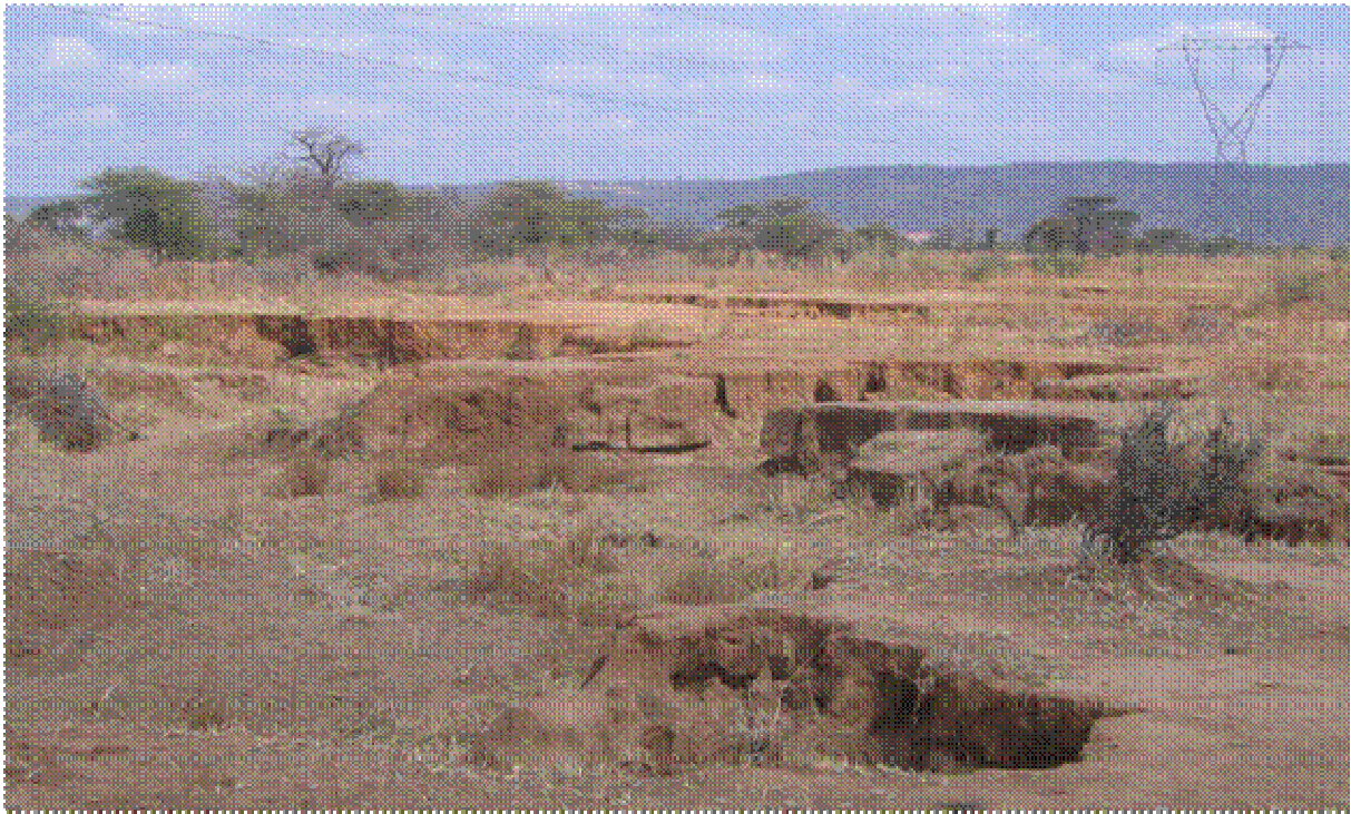
Figure 6-1: Soil Erosion (near Mlowa Barabarani)
