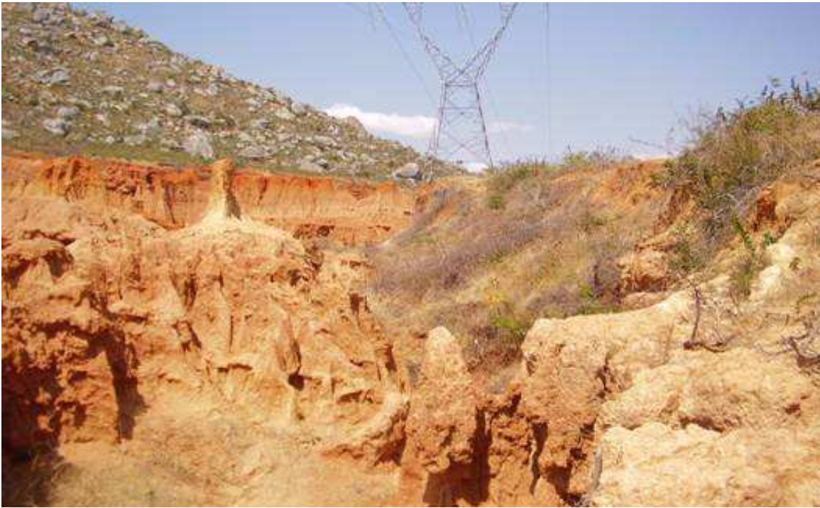
Figure 4-8: Tower Close to Erosion Prone Soil (Iringa Escarpment)
