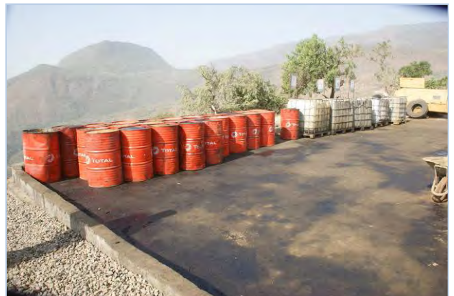
Fully bunded storage area for hazardous materials (oil and grease, Sika products etc)
