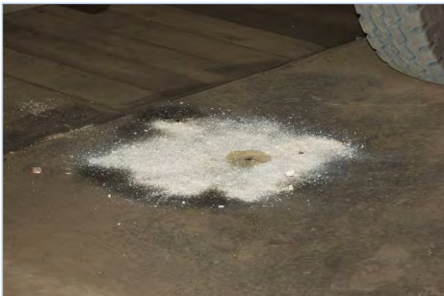
Use of absorbent material on oil spilled on the concrete ground
