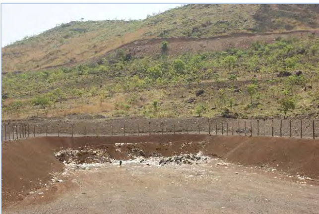
Central landfill for domestic solid waste. The bottom is covered by a compacted layer of clay.
