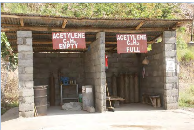
Waste water from the acetylene plant is collected...
