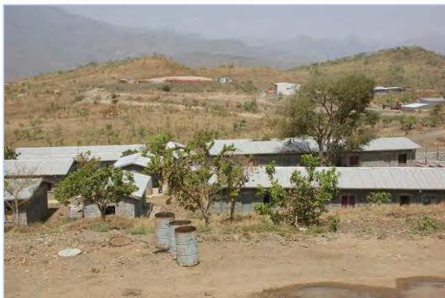
View of the left bank worker camp
