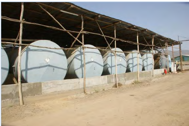
Fuel storage area with full concrete slab and bunds
