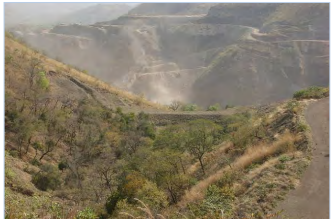
Lower part of Basalt Quarry No.2 where a weir has been built to avoid the transport of sediments from the site during the rainy season
