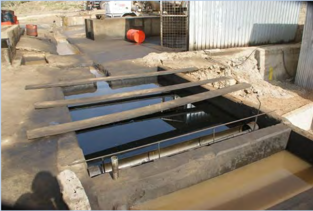
Water from truck cleaning & maintenance areas is collected and treated: oil separation by skimming, sedimentation then....
