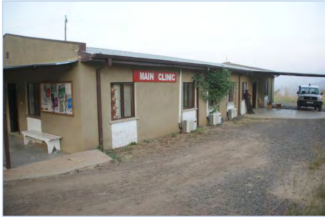
Three clinics (EPC Contractor camp, 2 worker camps) and 2 first aid posts (Offices and Power House) have been built (Picture: right bank worker camp clinic)
