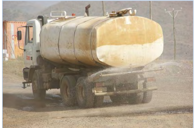
Watering of roads to reduce dust
