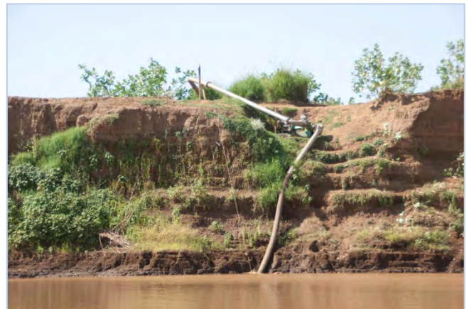
Motor pump along the Omo
