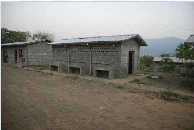
One sanitary block per every 2 buildings of 8 rooms each. Each block includes 6 washbasins (24 taps), 9 showers and 5 toilets
